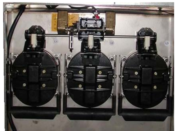
Detail of fuse holder inside the cell
